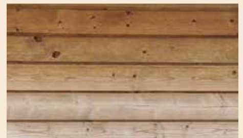
The wall of a brown dipped cabin that has been outdoors for four years without additional finishing. The part exposed to the sun is heavily faded.
