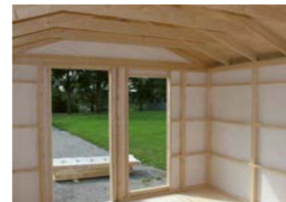
Internal view, walls covered with wind-protection plastic
