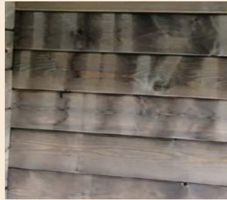
Colour variations caused by spacer bars
