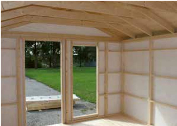
Internal view, walls covered with wind-protection plastic
