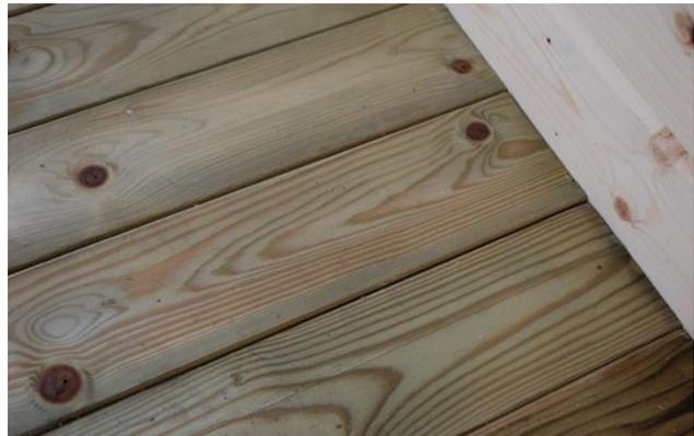
**TERRACE** – made from 28 x 120 mm terrace boards, green pressure treated.
